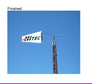
Model Engines have supplied us with a smaller Multiplex windsock so I have made a 4 metre high post that is hinged at the base so that the windsock can be replaced at ground level. This windsock is located beside the directional mustang and now it will be much easier and safer to glance sideways to see wind direction when landing, rather than looking back to the original windsock.
