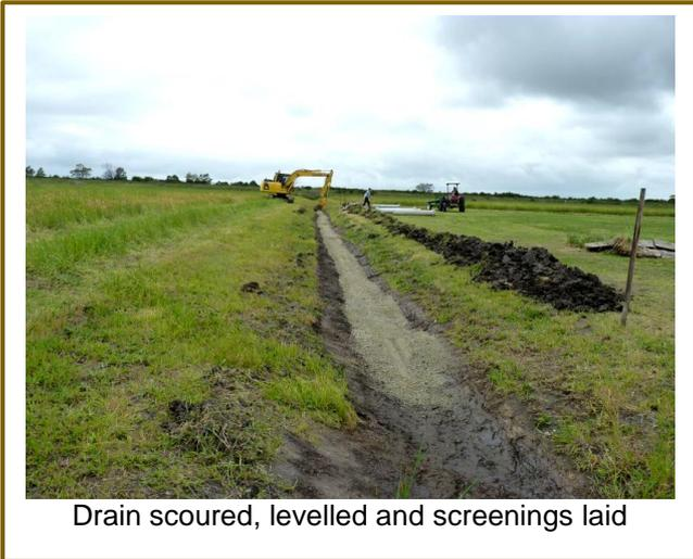
Drain scoured, levelled and screenings laid
