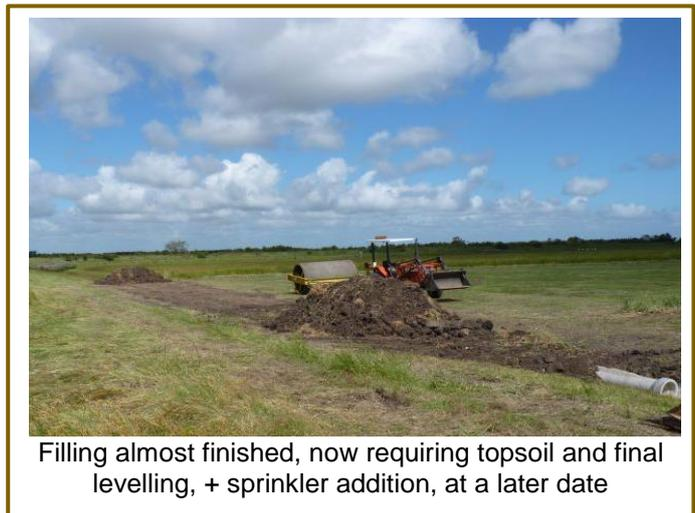
Filling almost finished, now requiring topsoil and final levelling, + sprinkler addition, at a later date
