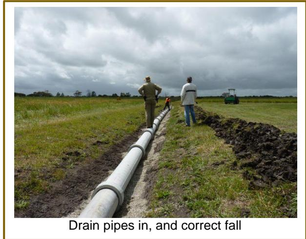
Drain pipes in, and correct fall
