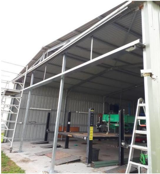
New top purlin + roof support posts bolted to the slab
