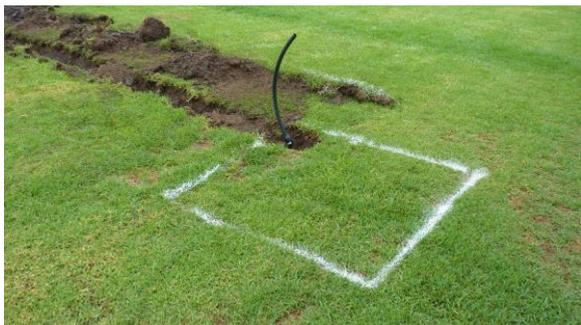
The new pipeline surfacing in the western pits area. The square is marked out for installation of a pit and electric pump, to help drain a troublesome wet area.
