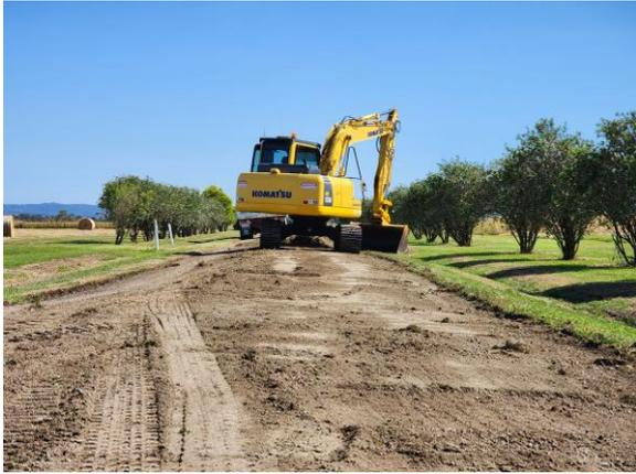
Cleaning up the edges of the driveway almost ready for adding crushed rock and topping.
