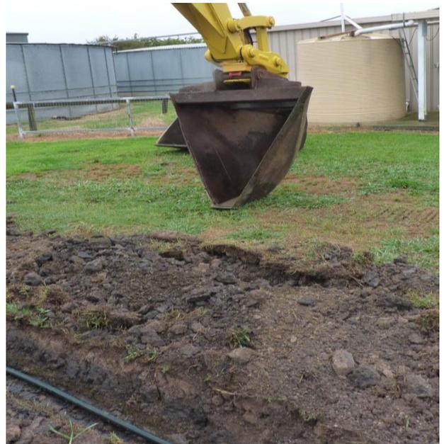
Glenn's trenching bucket plus the trench with the New pipeline laying in it. This bucket made short work of what would have been hours of work for us.
