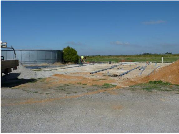
Laying out the trusses, and bolting them together
