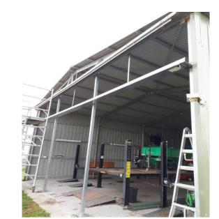
New top purlin + roof support posts bolted to the slab
