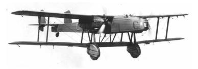
the fuselage, definitely not the norm! The undercarriage was streamlined with huge fairings which looked very utilitarian to put it politely. They were in fact utilitarian in that they did reduce drag by a remarkable amount and enclosed the fueling and oiling points which made servicing the aircraft so much easier than others.
