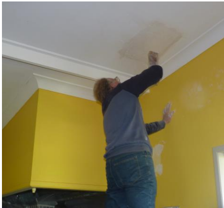
Peter Harris sanding ceiling filler
