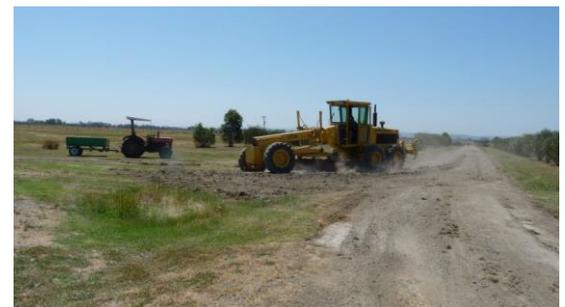
The graded rubble was used as fill for a low section near the start of the road to the western car park
