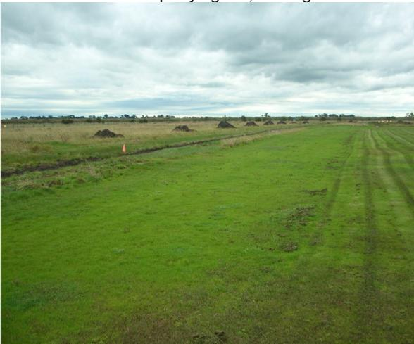
Main Strip drain looking West, this drain is designed to flow East and West from the centre of the Strip, laser graduated
