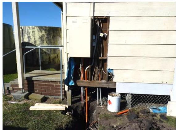
The shed cable in the bright orange conduit, going to the main switchboard
